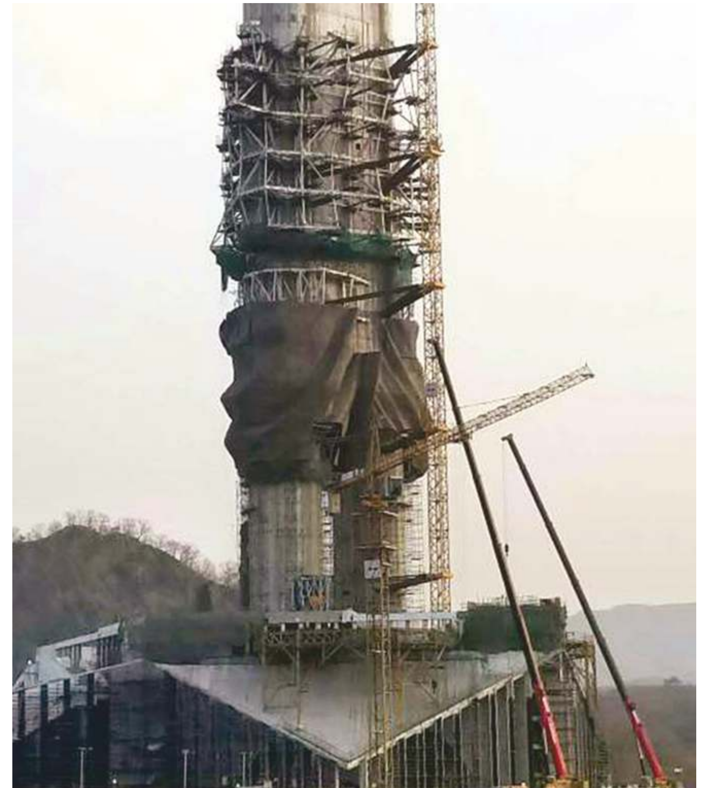
Bronze panels being installed on the core at site
