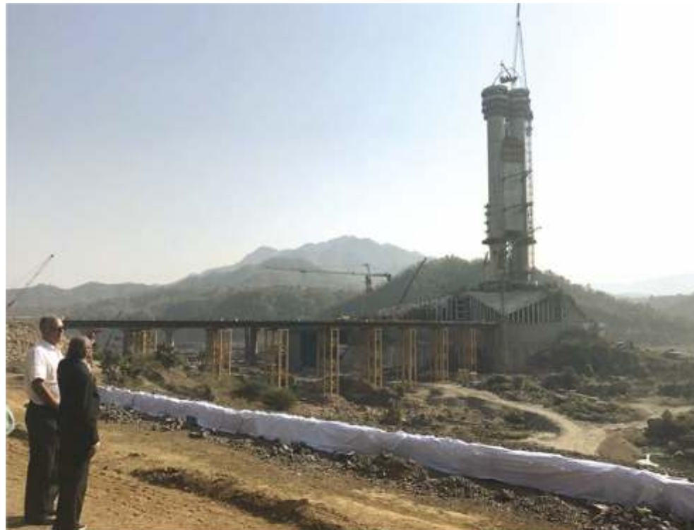
Completed concrete core at Sadhu Bet site & ready for installing Bronze panels
