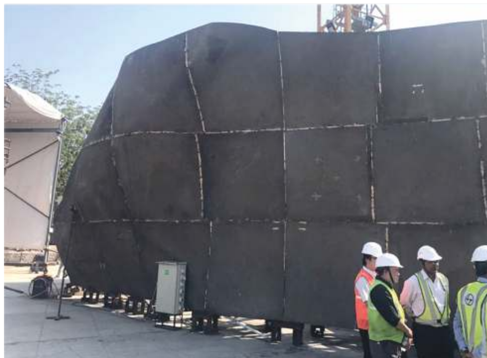
Final welding of Bronze panels at Sadhu Bet site
